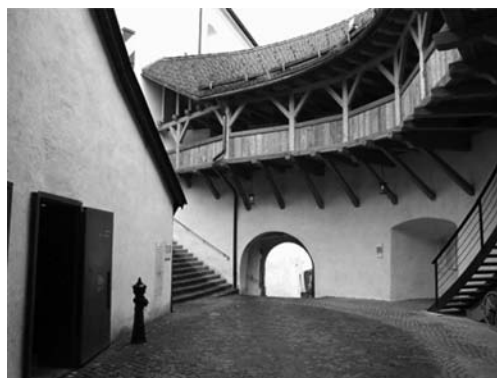
Figure 27.21. Digital photo of interior yard. (see colour plate page 509)
