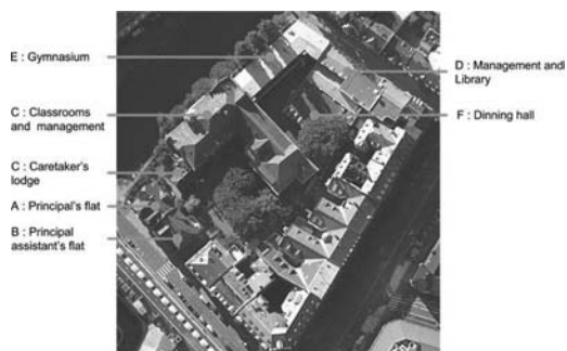
Figure 27.14(b). Aerial view of the site. (see colour plate page 506)
