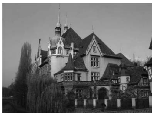
Figure 27.14(a). Overall view of the main building. (see colour plate page 506)
